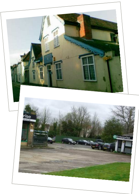
Top: The former British Legion building Above: Site of the proposed car wash
